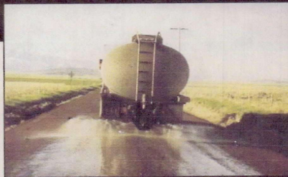
Truck spreading magnesium chloride for dust control
